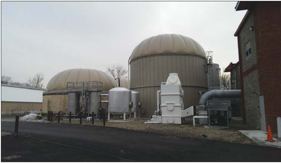
Figure 3. Phased Digestion and Gas Cleaning at Hermitage Municipal Authority
