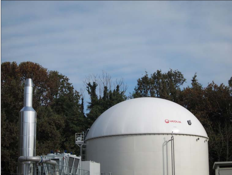
Figure 5. Veolia's Net-Positive Project in Lodi, Italy, Supplies Biomethane to Pipeline
